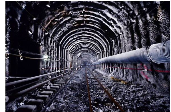
vertical shaft done: 400/600 m Sloped tunnel done: 950/1300 m
